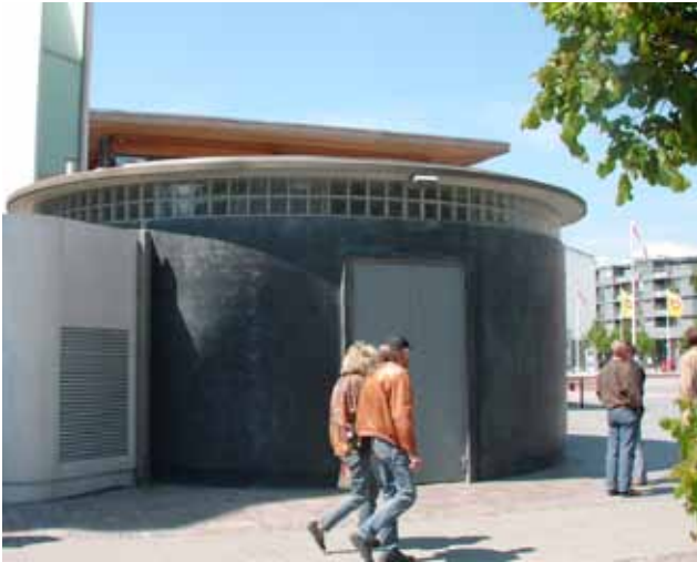
Pumpstation (Sundstorget Helsingborg)
